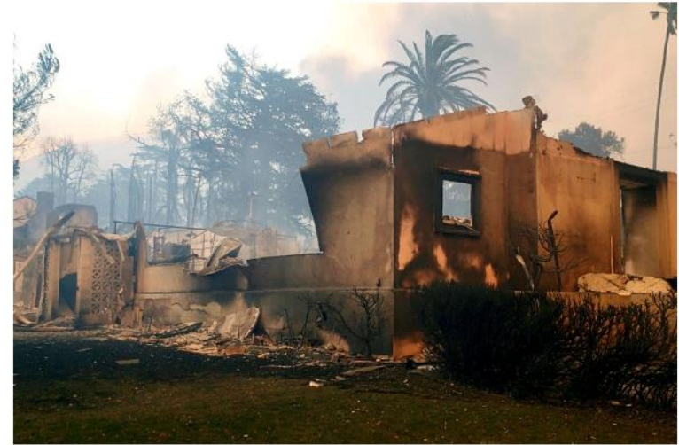
Altadena United Methodist Church in Altadena, Calif., is reduced to rubble after the Palisades and Eaton fires swept through Southern California. Experts warn that Los Angeles is not yet out of danger as the fires remain uncontained. Photo by the Rev. Garth Gilliam, district superintendent, California-Pacific Annual Conference.
